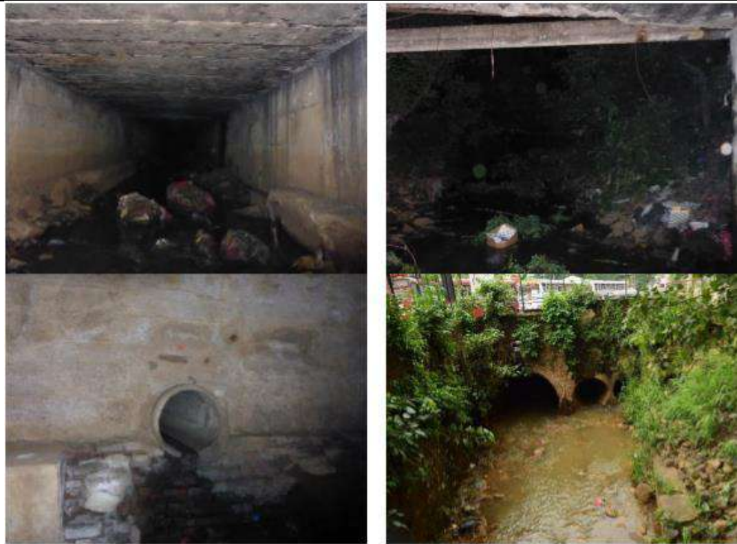
Fig. 4.12 Views of Medaela underground area at KMTT main Building site
