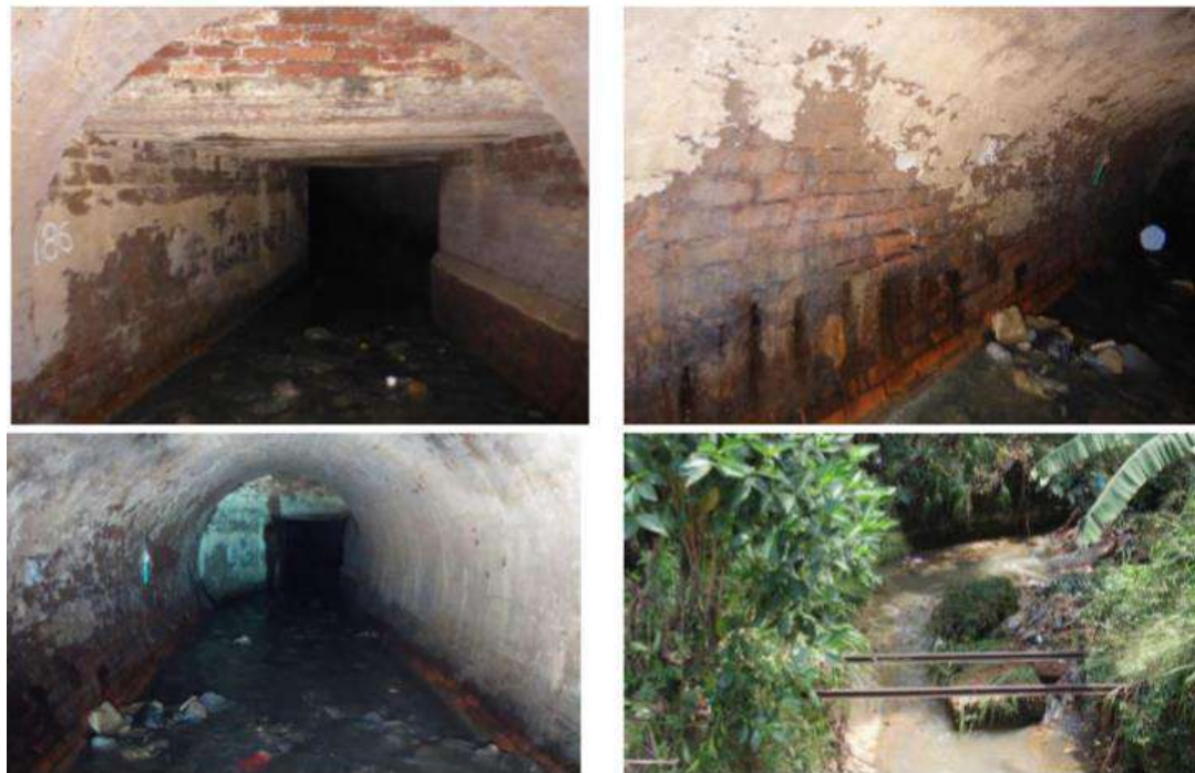
Fig. 4.10 Views of Medaela underground area at Railway Building site
