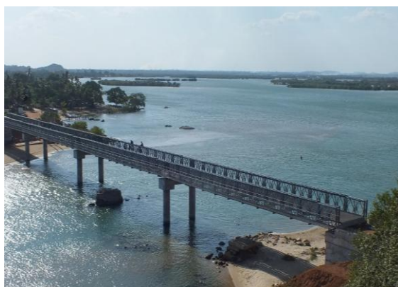
Lankapatuna Bridge on Sampoor Verugal Road
