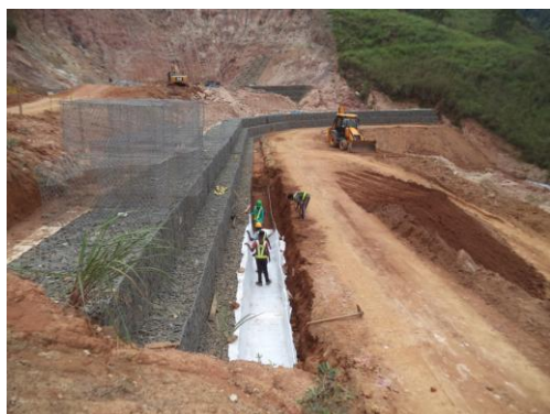
Geotextile laying for surface drain at Nuwara Eliya District
