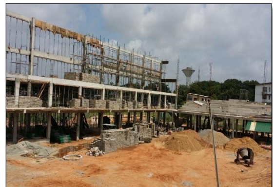
Fitness Centre University of Jaffna TEC Rs.. 242 Mn - Physical Progress 59%
