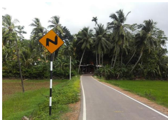
Sign Board Arrangement & Road Marking at Jaburegoda- Heelegoda Road
