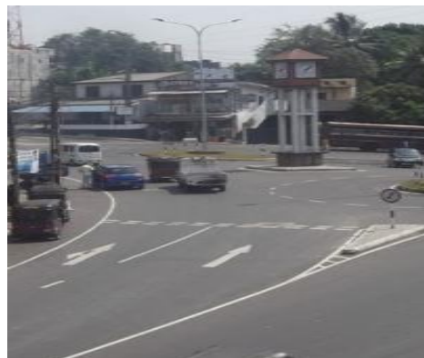
Welikada - Kohilawatta Road at IDH Junction
