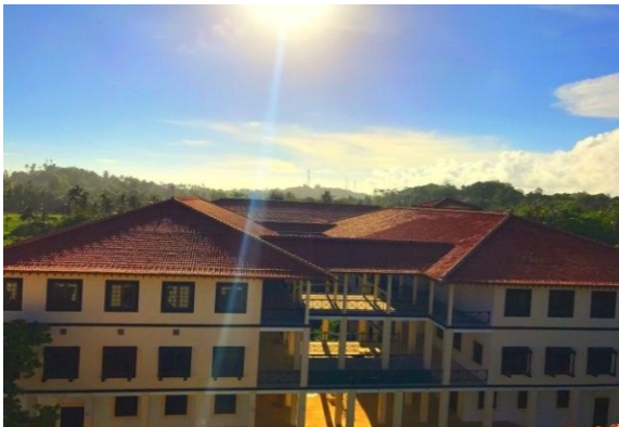
Three buildings for Faculty of Fisheries and Marine Sciences (Stage 11 ) – University of Ruhuna TEC Rs. 694.4 Mn
