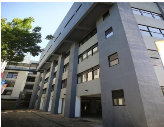
Extension for the East Wing of the building of the Faculty of Management & Finance - University of Colombo TEC Rs.. 130 Mn
