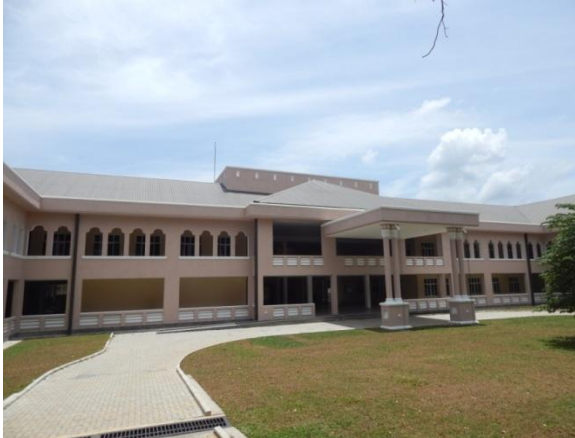
Project of Developing Faculty of Agriculture Stage 1 – University of Peradeniya TEC Rs. 930.4 Mn
