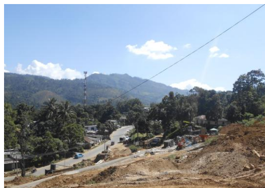
Progress of Earth works at Nuwara Eliya District
